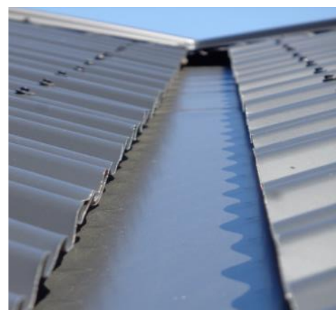
Example of finished Box Valley
