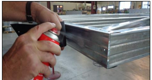
Gluing DPC to the Bottom Plate
